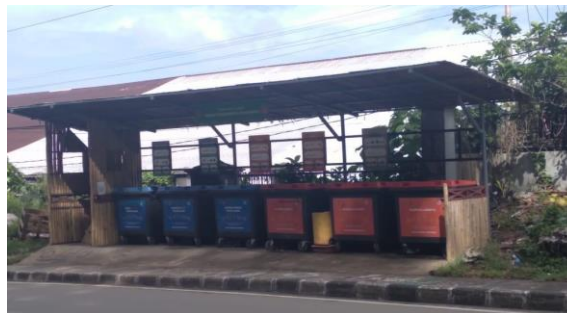
Figure 3. Waste Collection Point
