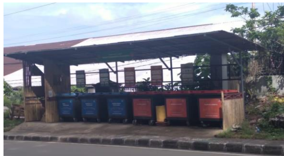
Figure 3. Waste Collection Point
